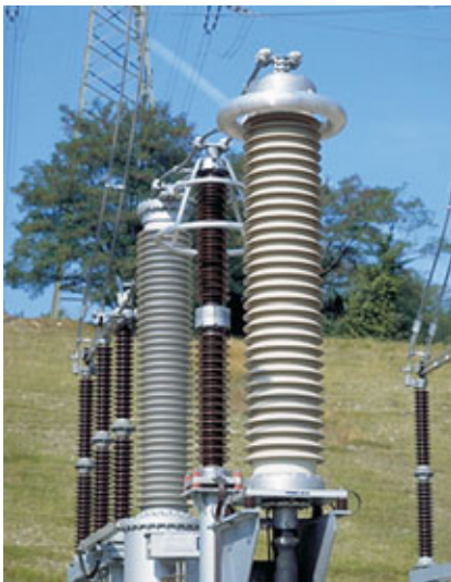
Picture 2 Outdoor termination 123...145 kV with composite insulator
